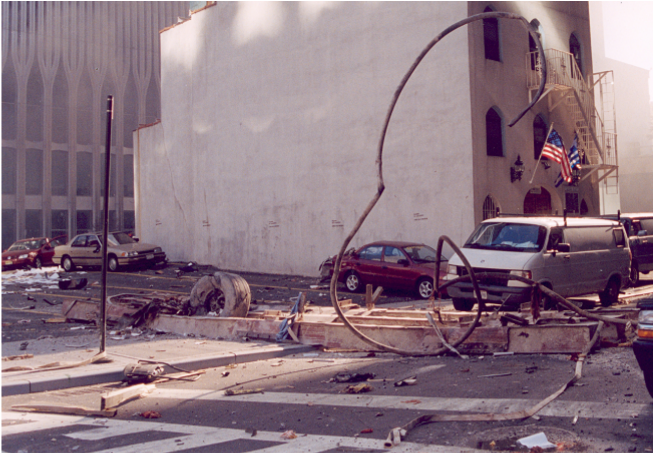
An exterior column section from WTC 1 with an embedded airplane wheel, beside St. Nicholas Church on Cedar St. at West St. WTC 2 is in view. NYPD photo , cropped (from 911datasets.org NIST FOIA 09-42 release 8, Roll 3 #12)
